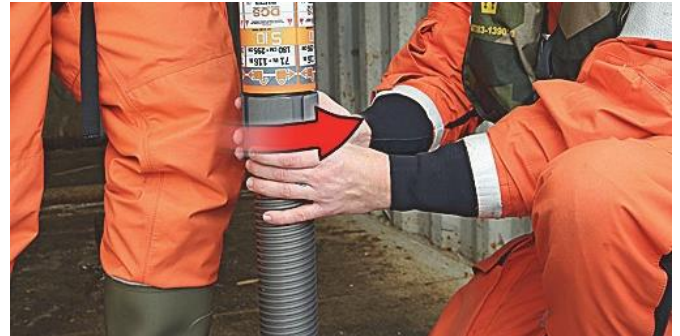
Figure 4-5: Adjusting the Shore
